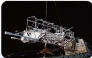
STEEL STRUCTURE FABRICATION
