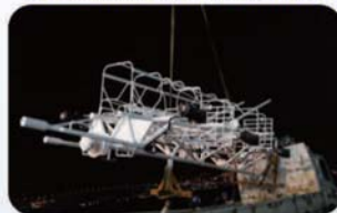
STEEL STRUCTURE FABRICATION
